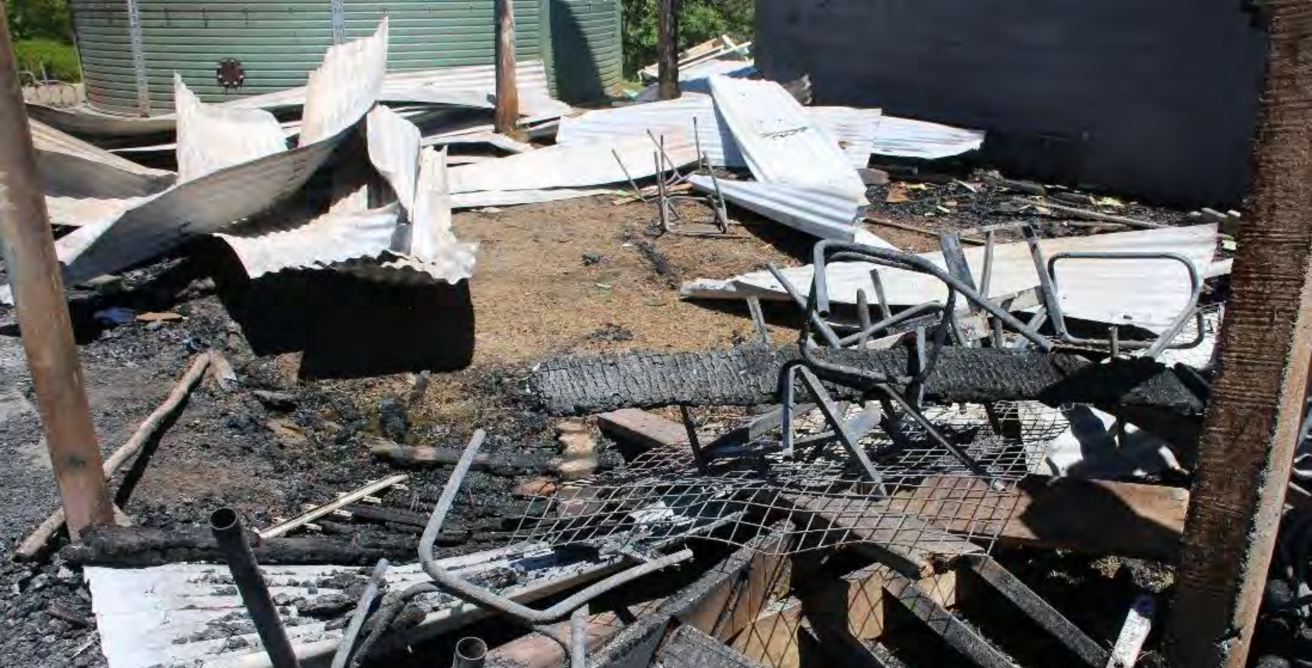
Burnt desks and chairs outside the building.
