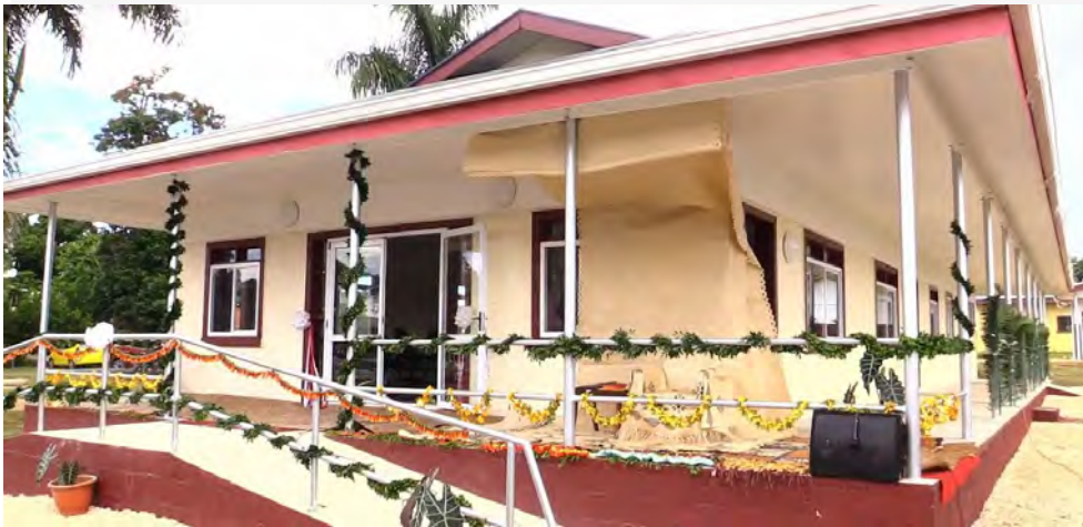
New Form 7 building
